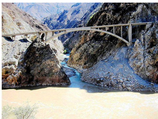
New bridge of Yunnan-Tibet Highway
